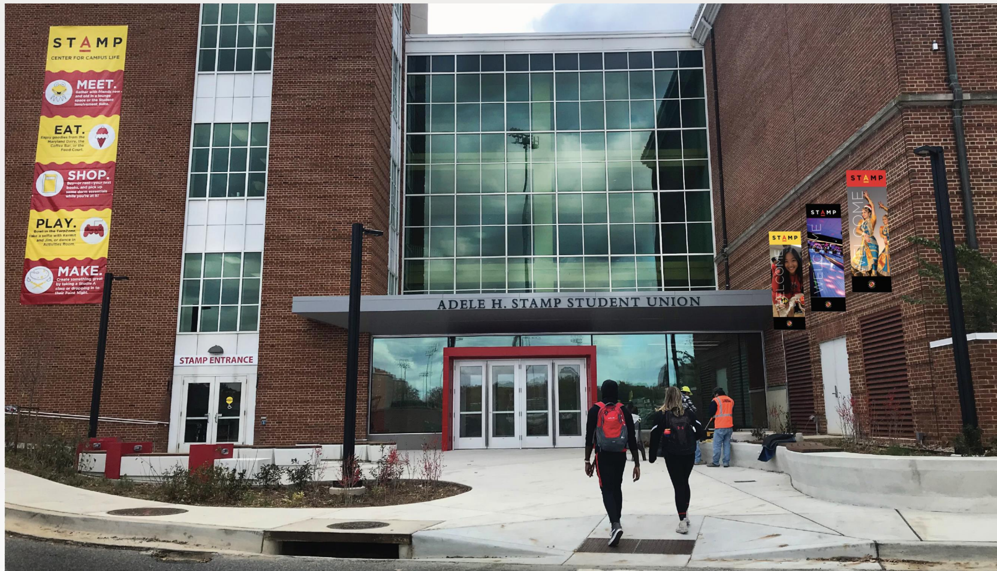
New North Entrance Project Completion at STAMP University of Maryland
